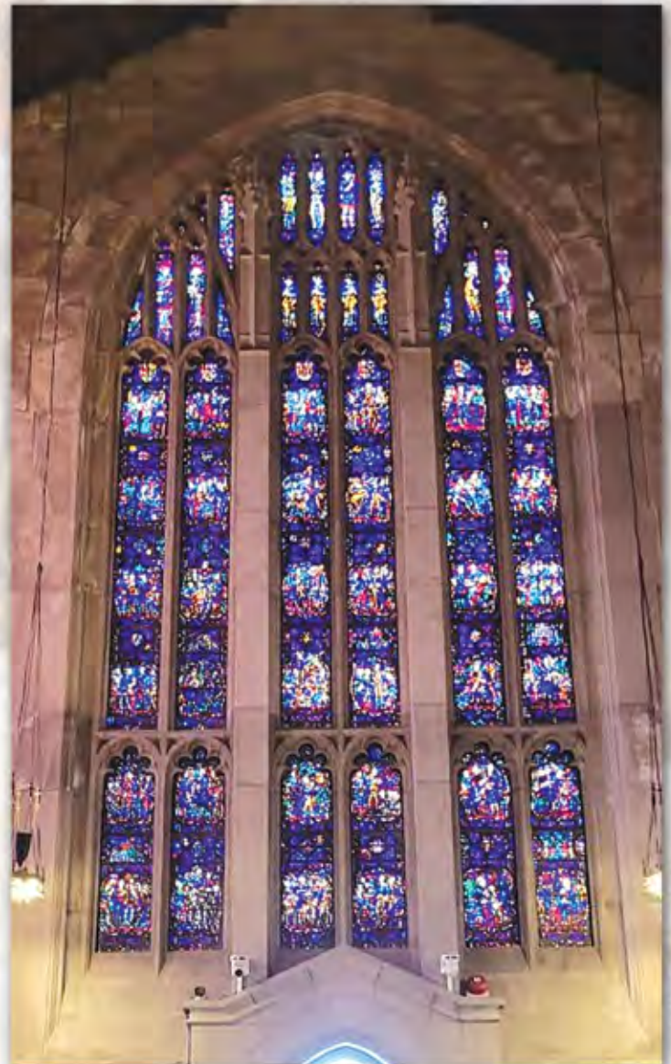
Interior view of chapel window prior to restoration.
