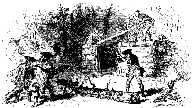
Felix O.C. Darley's 19th century depiction of the construction of log huts at Valley Forge.
